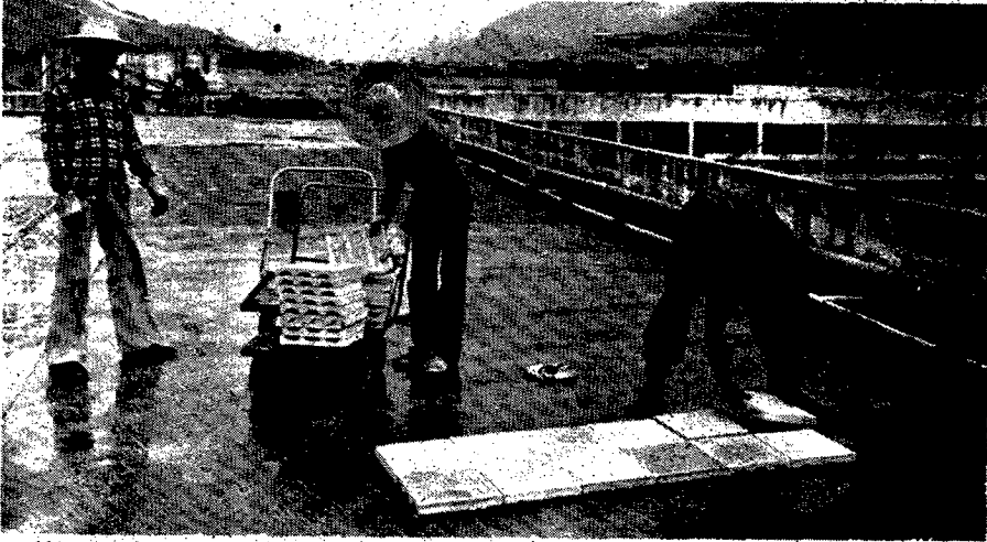
Workers laying lightweight insulation on the roof of a block at Upper Pak Tin estate where re-roofing is in progress.
